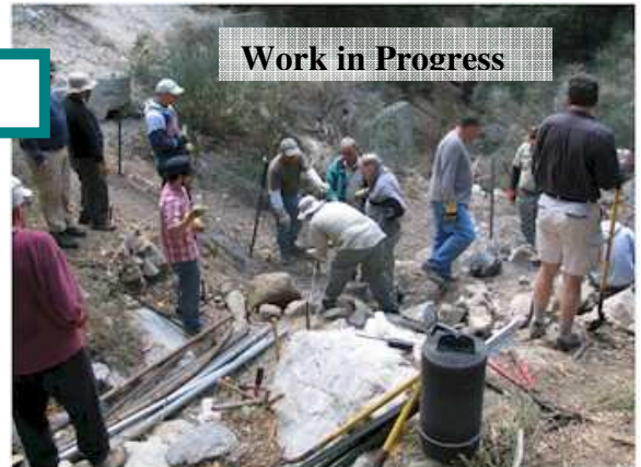
Debris dam assembly in progress.
